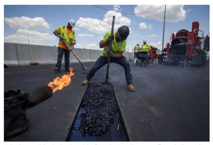
Workers heat, pound, shovel and cart hot asphalt to form a plug joint on the new ramp off I-91 to the Charter Oak Bridge and I-84 East. The work is putting the finishing touches on the new exit, which took a little over two years to build. (Mark Mirko/Mark Mirko)
