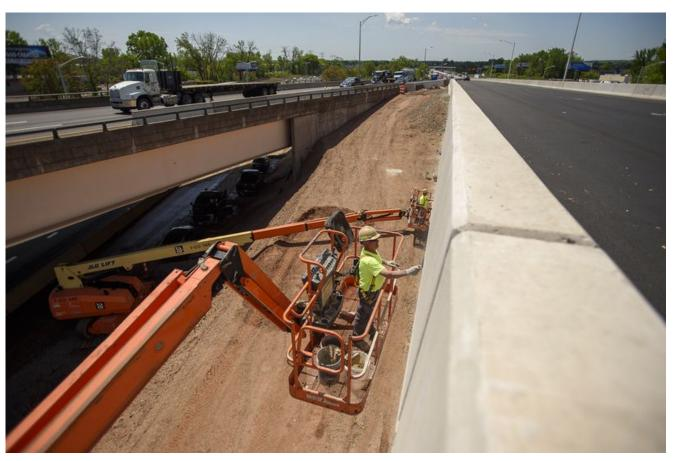
Workers finish concrete on the side of the new ramp off I-91 to the Charter Oak Bridge and I-84 East. The new ramp will open to the first travelers shortly after midnight on Wednesday. (Mark Mirko/Mark Mirko)
